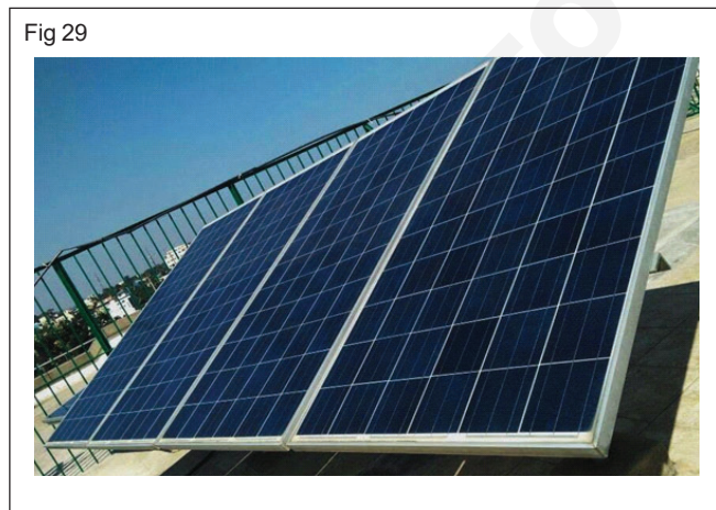
Solar panels 4 x 250 W mounted on mounting structures. (Fig 29)
